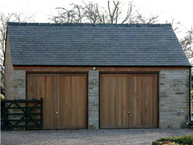
Typical Image: Courtyard and adjoining garage
